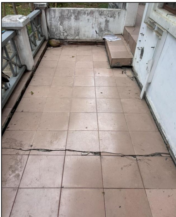
Figure 1.10 Settlement of Ground floor
