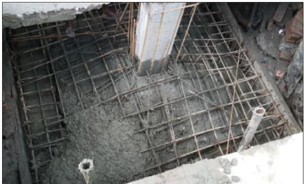
Figure 2.9 Strengthening of Footing
